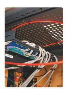
This system does not occupy valuable rack space and FDT can be run unobtrusively across the top of the rack
