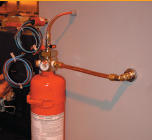
Mounted Firetrace system including pressure switches
