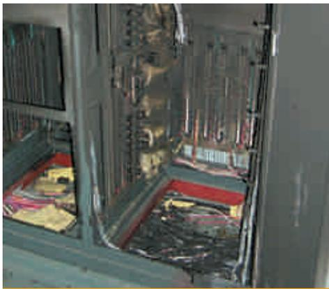
A small fire in a single cabinet, unchecked, can easily grow to consume adjacent cabinets - or even spread throughout a facility.
